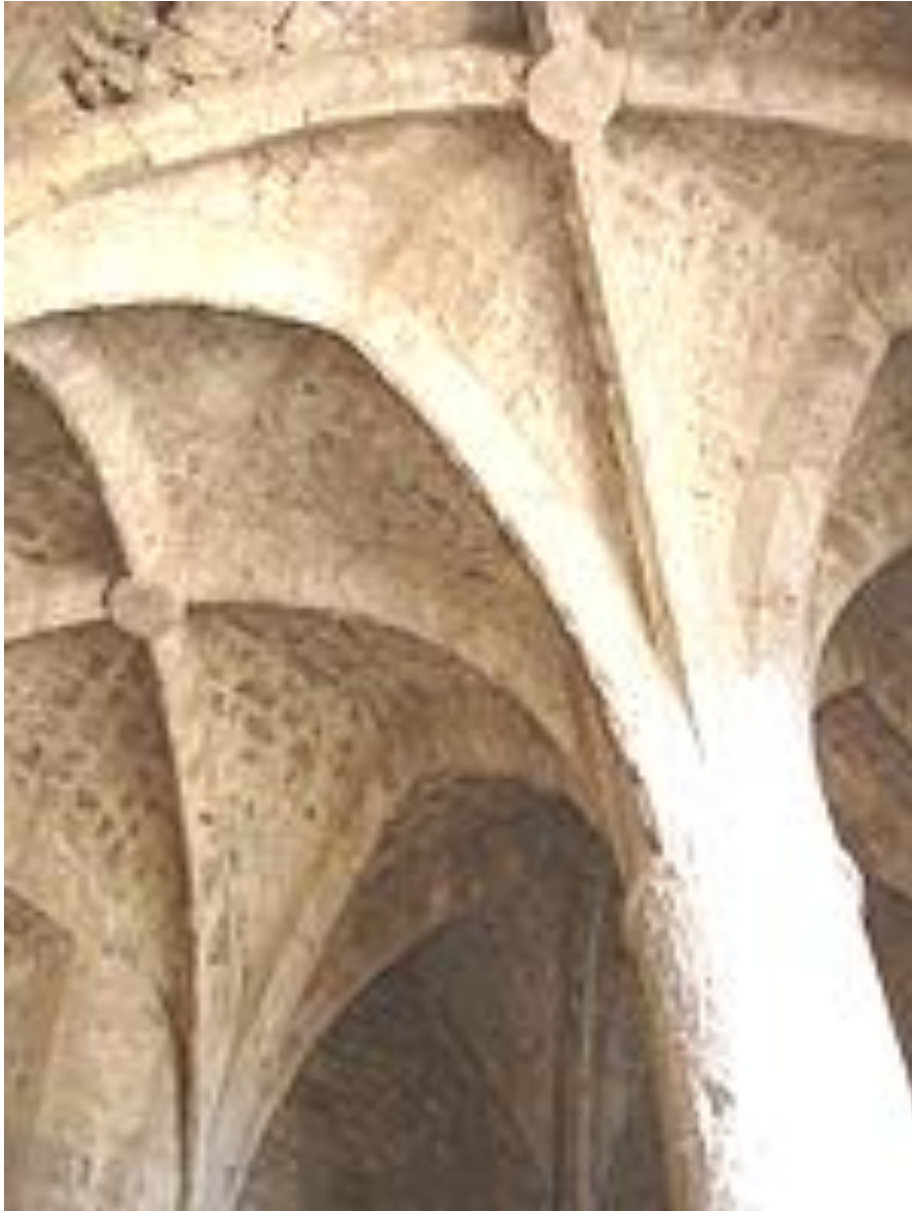
Cross-vault ceiling with keystone Château de Quéribus, France
