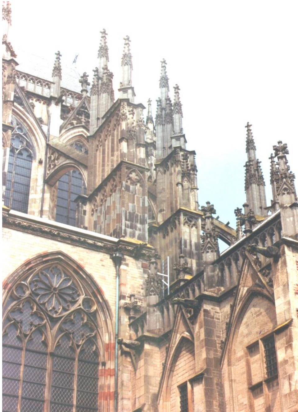
St. Martin's Cathedral, Utrecht, the Netherlands (built 1254 - 1517)
